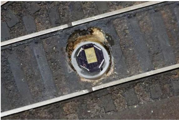
When installed, the detector will look like this. This was a retrofit, so it isn't as neat as an original installation will be.
